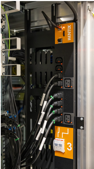
Kentix SmartPDU with RCM
