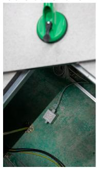
Kentix leakage sensor in raised floor
