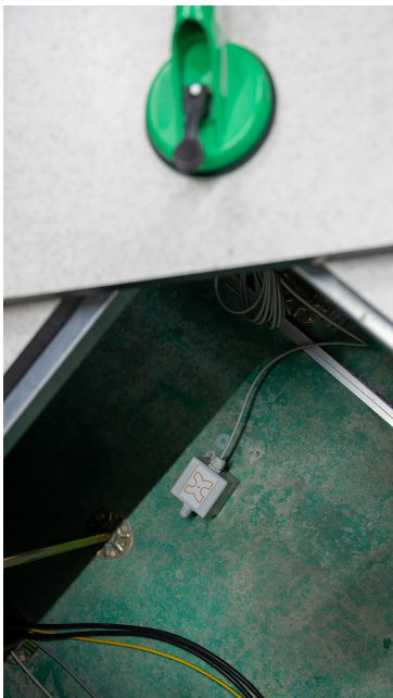
Kentix leakage sensor in raised floor
