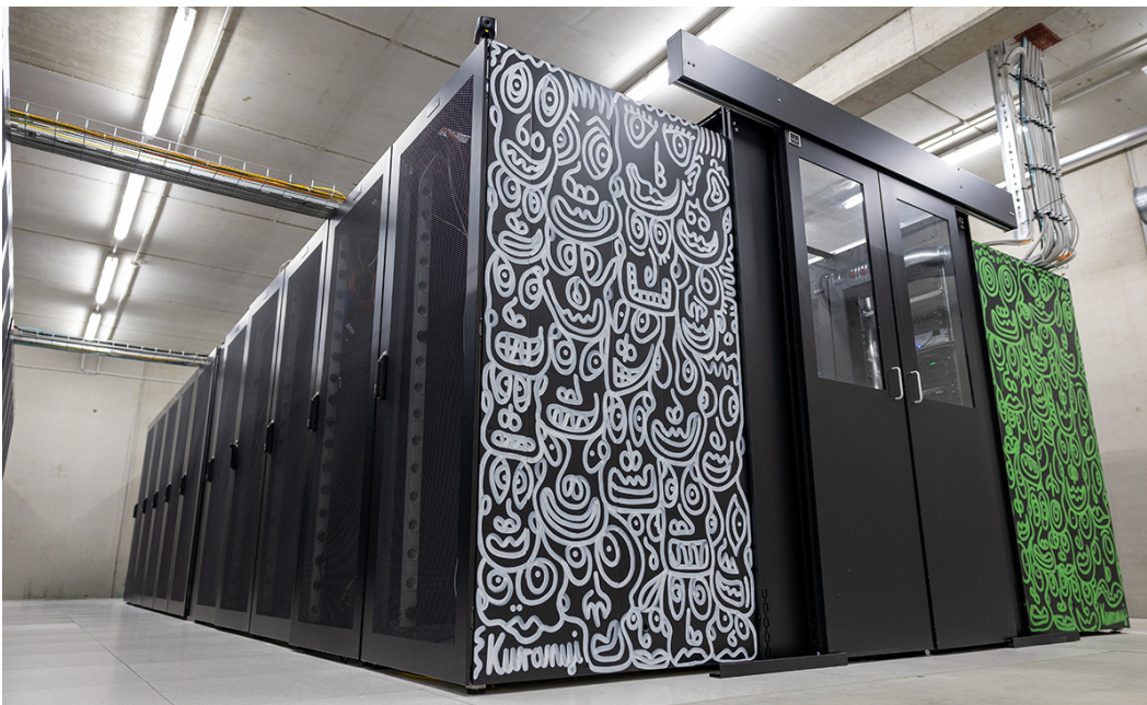
Cold aisle containment with seamless monitoring via Kentix MultiSensors and SmartPDU
