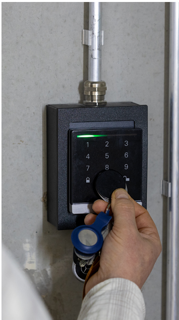
RFID wall reader with 2FA authentication
