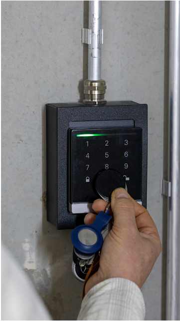
RFID wall reader with 2FA authentication
